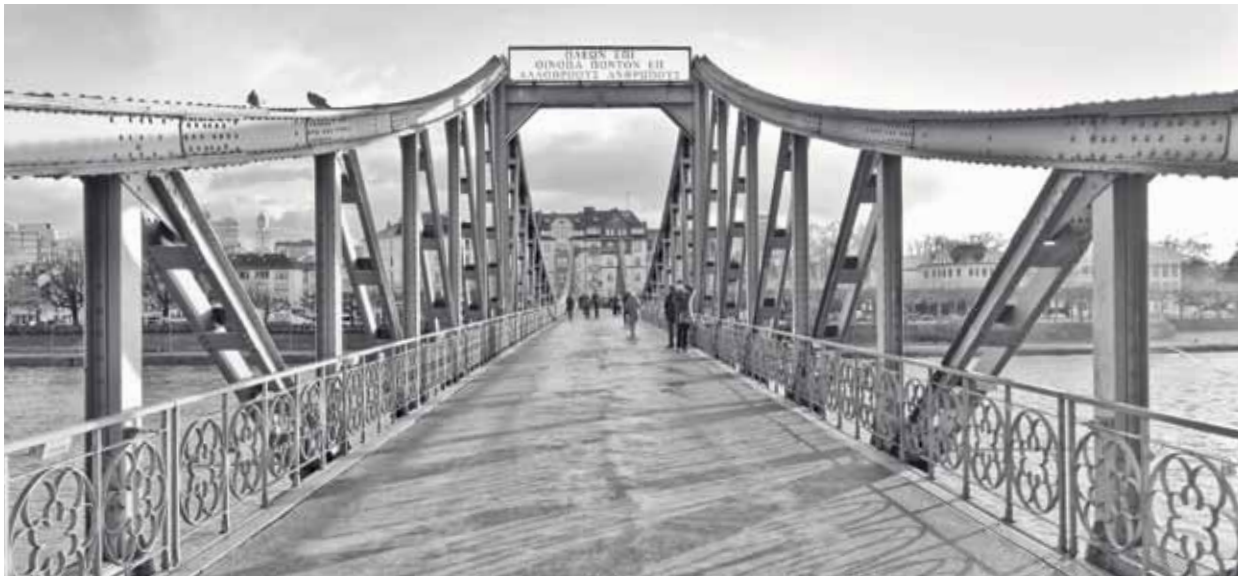
The Eiserner Steg steel bridge built in 1868 in Frankfurt, Germany
