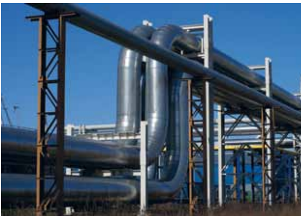
Industrial steel pipelines
