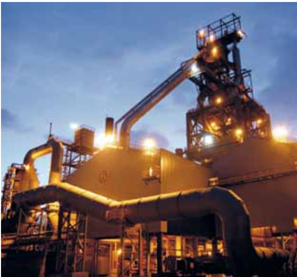
Number 5 Blast Furnace at the Port Talbot Tata Steel (formerly Corus) Plant in South Wales, United Kingdom
