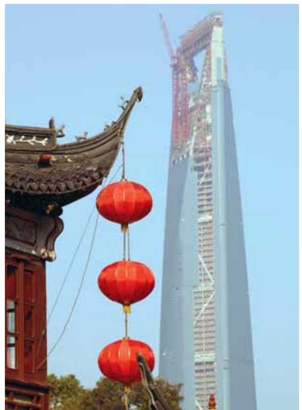
World Financial Center in construction, Shanghai, China (2008). The design, using a diagonal-braced frame, employs an effective use of material, because it decreases the thickness of the outer core shear walls and the weight of the structural steel in the perimeter walls
