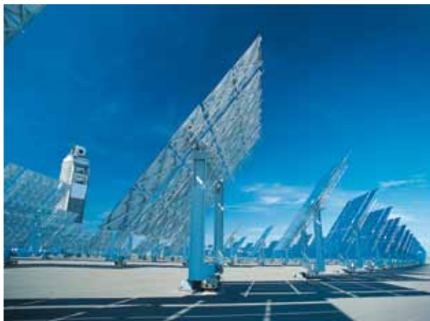
Solar power panels, Albuquerque, New Mexico, US. Steel bases are used to ensure the panels' strength and security
